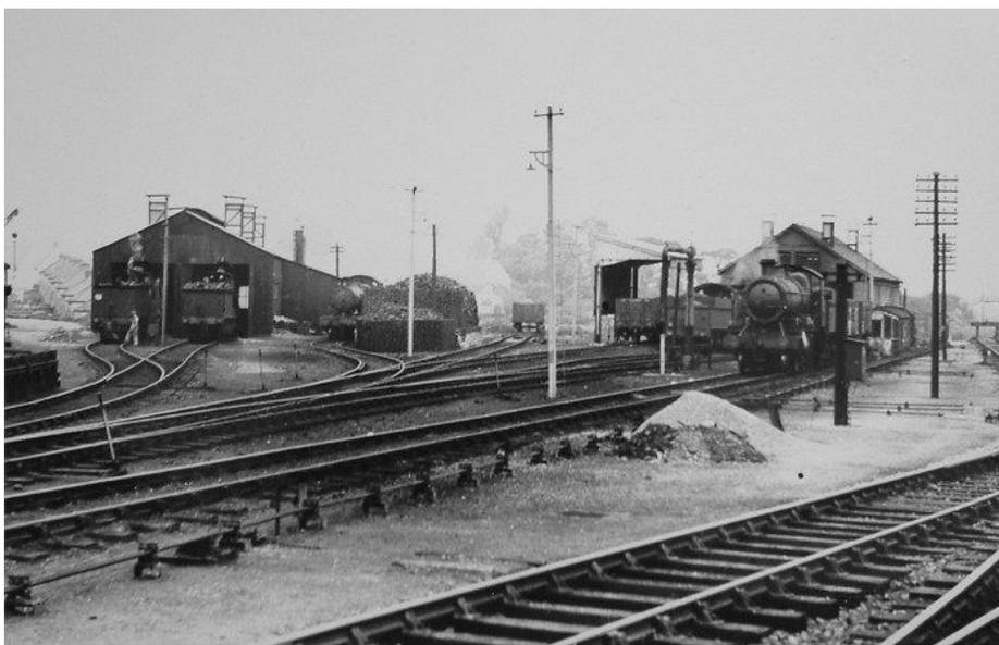
Very early photo of Andover Junction shed at a time when there were in fact two sheds, one for the MSWJR and the other for the SWR. When the regions were amalgamated in 1948 the two sheds were combined into one. At some point the shed on the right of the photo was demolished because in 1956 when I worked there only the engine shed on the left of the photo remained. Picture courtesy of your website
