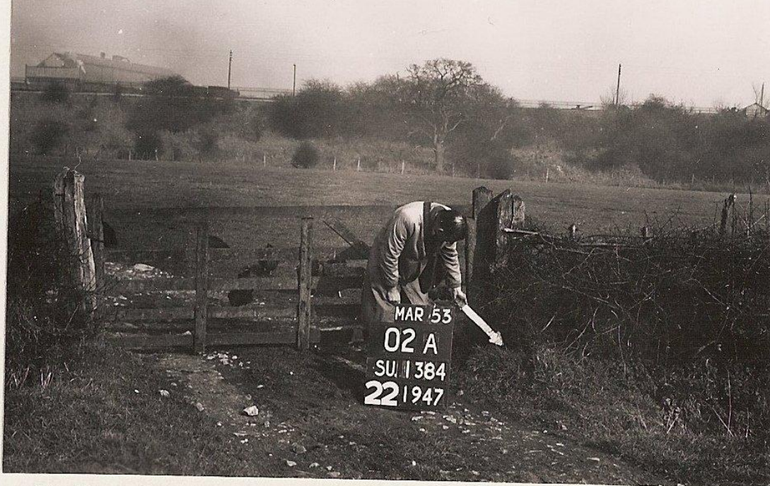
R.P. 02A. Pipe Nail in gate post.
